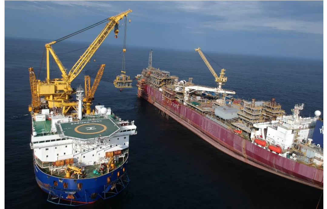
New gas lift compressor lifted on board BW Adolo
